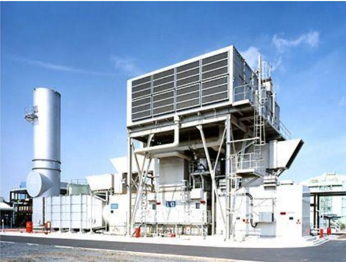
Simple cycle gas turbines began to penetrate the electric generation fleet in the 1960s. Early vintage gas turbines were relatively inexpensive to build on a \$/kW basis, but were inefficient and generally limited to smaller size units. Because of their inefficiency, they were limited to serving load only during peak load and emergency operating conditions (i.e. less than 1,000 hours per year).
